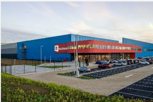
U.K. Flavor Solutions Manufacturing Facility
